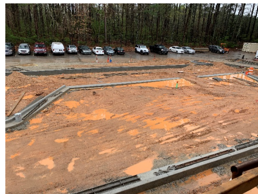
South Elevation Curb and Gutter
